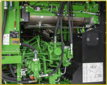
C. Clean door latch, auxiliary drive gear case, hydraulic pumps, and exhaust components.
