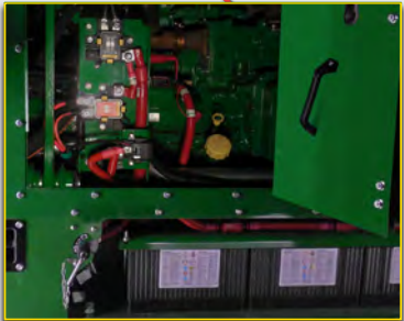
D. Clean rear of engine, turbocharger, exhaust manifold, starter, and battery area.
